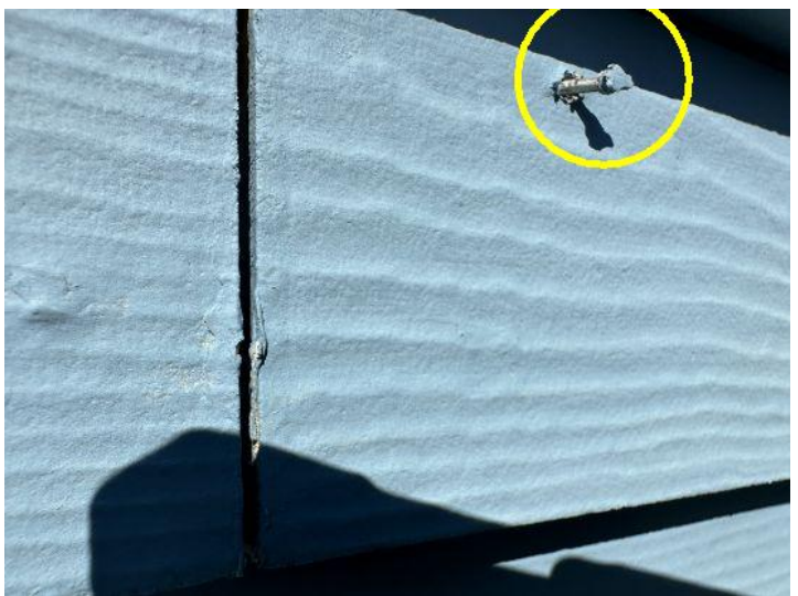
Cement siding (hardie board) has several nail pops; recommend re-nailing and sealing as needed.
