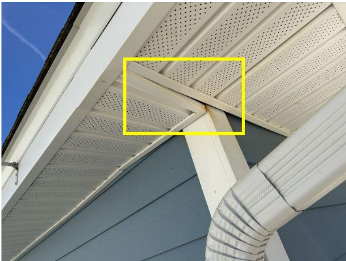
Vinyl soffit is loose on the front left corner.
