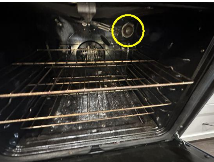
Oven light not working; possibly a bad light bulb.
