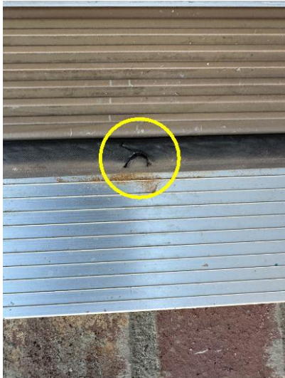
Small tear in the weather stripping along the bottom of the back door.
