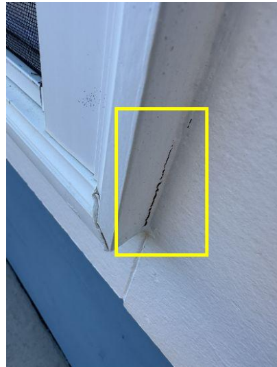
Recommend sealing/caulking around window and door frames as needed to prevent moisture intrusion.
